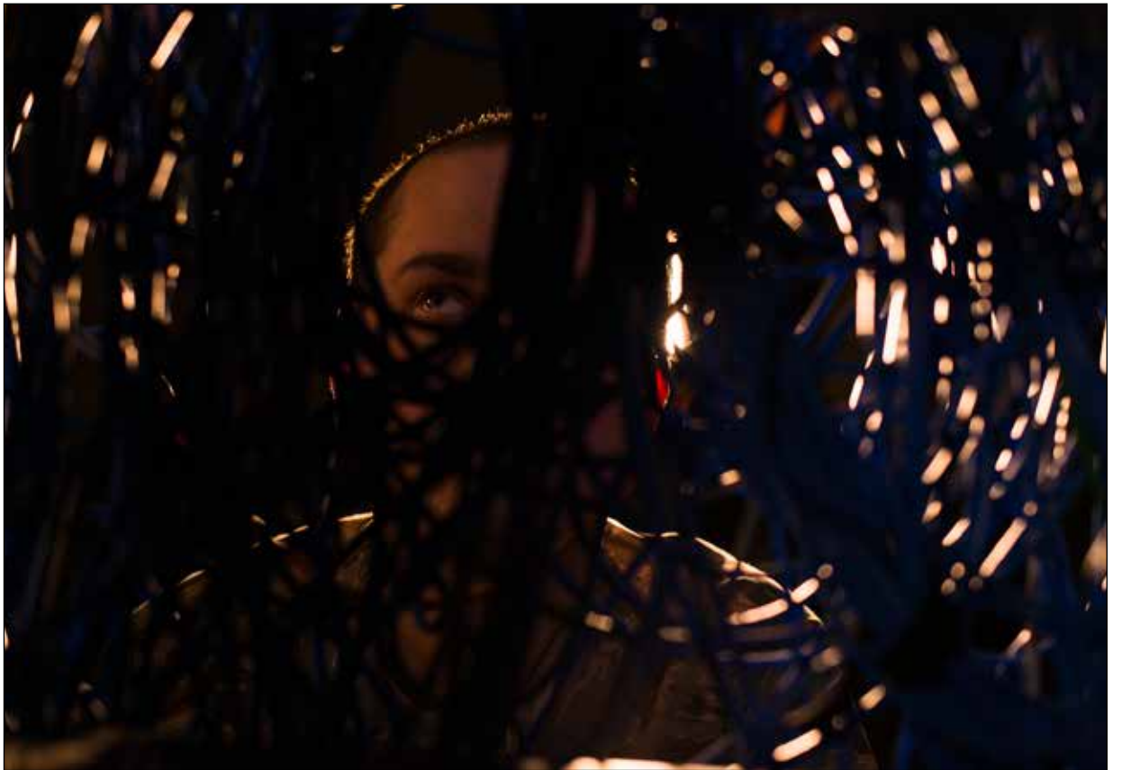
Senior Airman Neil Kenny, 51st Communications Squadron client systems technician, looks through wires into a switchboard Feb. 10, 2015, at Osan Air Base, Republic of Korea. Kenny is one of 34 CSTs who provide service for more than 7,000 customers on base. (U.S. Air Force photos by Senior Airman Matthew Lancaster)
