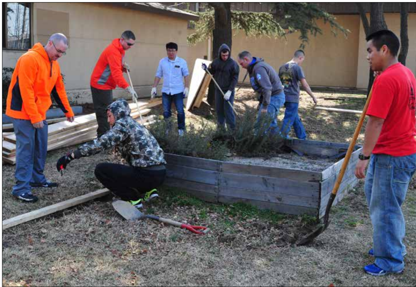
8th Fighter Wing Airmen build the foundation for "Wolf Pack Garden" in front of the Sonlight Inn, March 14, 2015, at Kunsan Air Base, Republic of Korea. The garden is part of a community initiative to promote healthy living for Wolf Pack Airmen. (U.S. Air Force photo by Capt. Reba Good)
