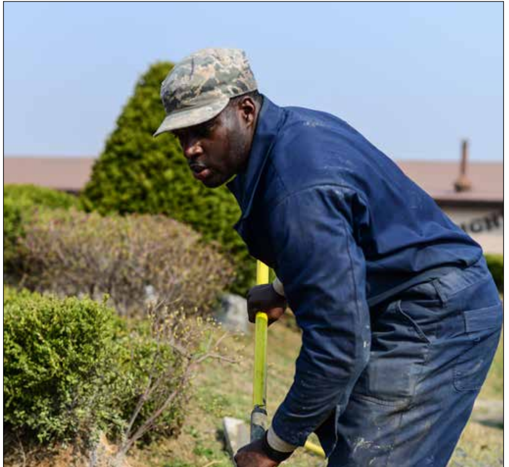
Staff Sgt. Ernest A. Opoku, 51st Civil Engineering Squadron Pavement and Equipment Operator, spreads concrete April 10, 2015, at Osan Air Base, Republic of Korea. Individuals who are chosen for this spotlight recognition are distinguished as consistent, superior performers within their squadrons. (U.S. Air Force photo by Senior Airman Matt Lancaster)
