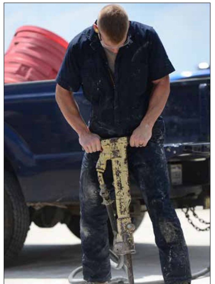
Airman 1st Class Zachary Downing, 51st Civil Engineer Squadron pavement and construction equipment apprentice, jackhammers out a broken section of pavement before the mixing, pouring, and finishing of the new concrete patch can begin on the airfields of Osan Air Base, Republic of Korea, June 27, 2015. As a member of the group known as the "Dirt Boyz," Downing is trained to operate a vast array of heavy machinery.
