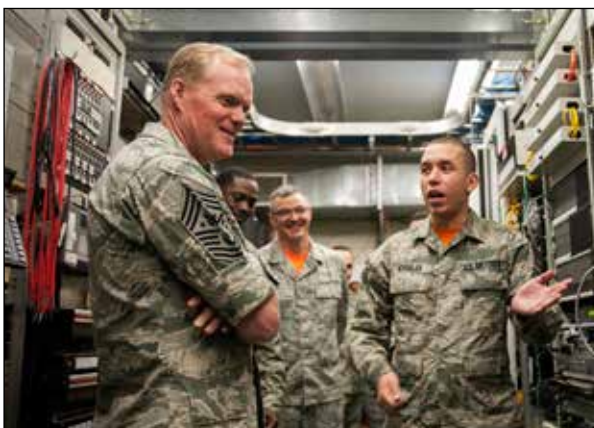
Senior Airman Luis Morales, 8th Communications Squadron technician, explains the Wolf Pack's main circuit structure to Chief Master Sgt. of the Air Force James A. Cody at Kunsan Air Base, Republic of Korea, July 3, 2015. Cody met with Airmen from the 8th Fighter Wing during his second visit to Kunsan July 2 and 3 to see first-hand how the Wolf Pack trains to defend the base, accept follow-on forces and take the fight north. (U.S. Air Force photo by Senior Airman Katrina Heikkinen)
