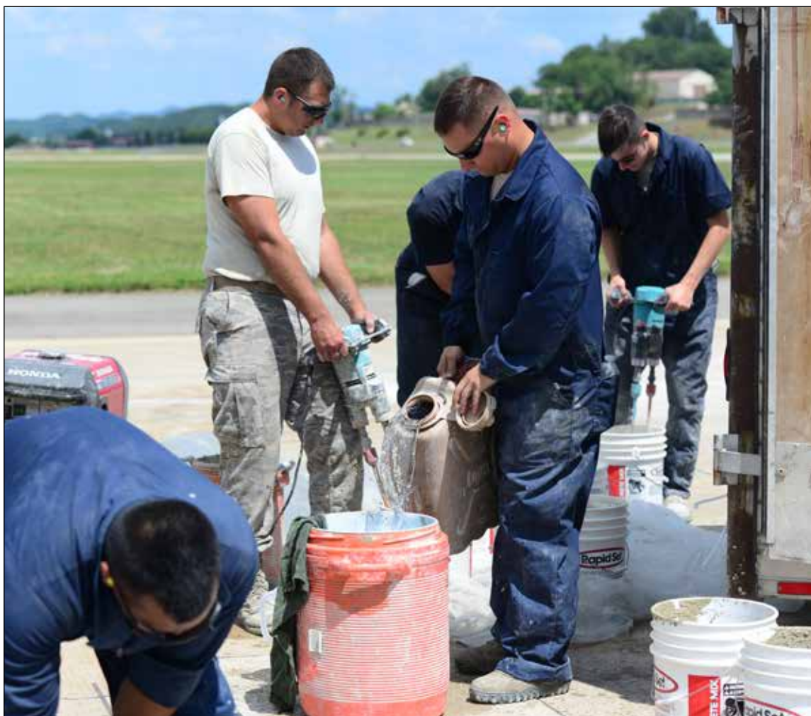
Airmen from the 51st Civil Engineer Squadron pavement and construction equipment shop, also known as the "Dirt Boyz," perform spot repairs on sections of the airfields at Osan Air Base, Republic of Korea, June 27, 2015. Since January 1, 2015 the "Boyz" have logged over 3,000 man hours completing more than 2,000 such repairs on the 1.5 million square yards of Osan's airfield.
