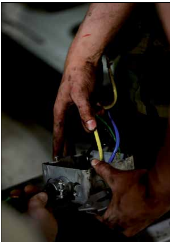
Airmen of the 51st Civil Engineer Squadron heating, ventilation and air conditioning shop work to repair the wiring in a dormitory unit at Osan Air Base, May 13, 2015.
