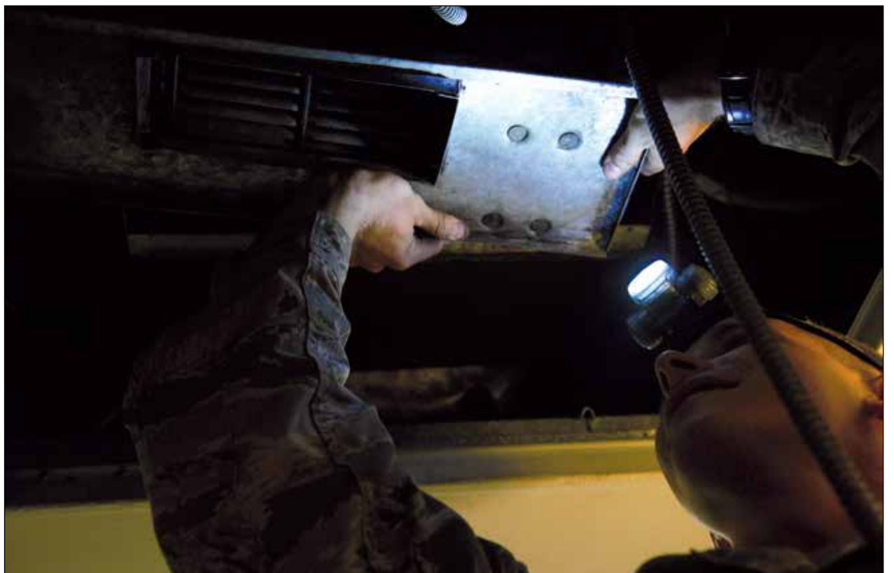
Airman 1st Class Evan Evans, 51st Civil Engineer Squadron heating, ventilation and air conditioning/refrigeration apprentice, works to replace the fan in a dormitory room at Osan Air Base, July 10, 2015. Evans is part of the skilled team of technicians that keep Osan's air running year round.
