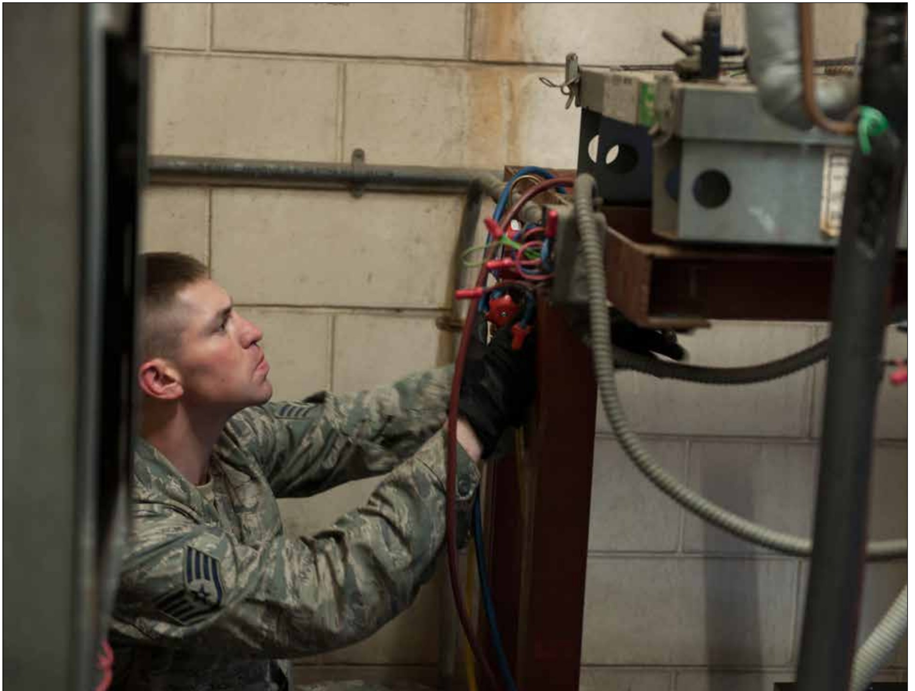
Staff Sgt. Matthew Browning, 8th Civil Engineer Squadron Heating, Ventilation, Air Conditioning and Refrigeration shop craftsman, sets up the condenser for the dining facility at Kunsan Air Base, Republic of Korea, Sept. 4, 2015. (U.S. Air Force photos by Senior Airman Dustin King/Released)
