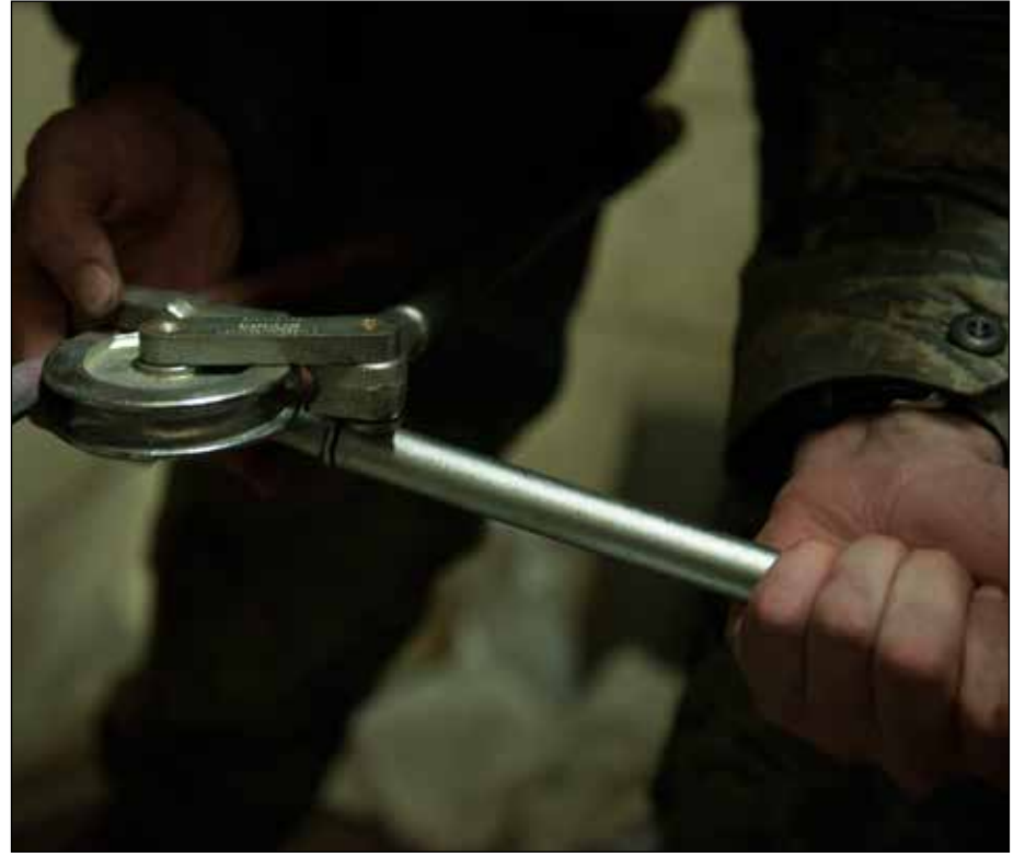
Staff Sgt. Matthew Browning, 8th Civil Engineer Squadron Heating, Ventilation, Air Conditioning and Refrigeration shop craftsman, measures out copper to bend and form to the condenser, at Kunsan Air Base, Republic of Korea, Sept. 4, 2015. HVAC-R Airmen are responsible for installing, and repairing heating, ventilation, air conditioning and refrigeration units.
