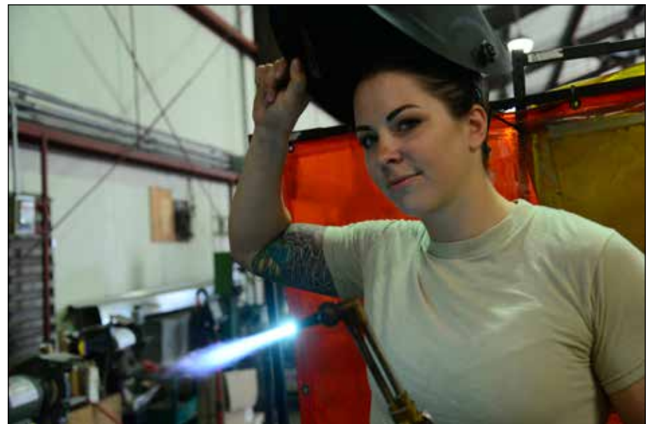
Staff Sgt. Bethanie Jeremenko, a 51st Civil Engineer Squadron structural craftsman, proudly poses holding one of her favorite tools, an industrial blow torch at Osan Air Base, Republic of Korea, July 30, 2015. Whether cutting, painting, welding or building, no job is too big or too small for an Airman of the 51st Civil Engineer Squadron structures shop.
