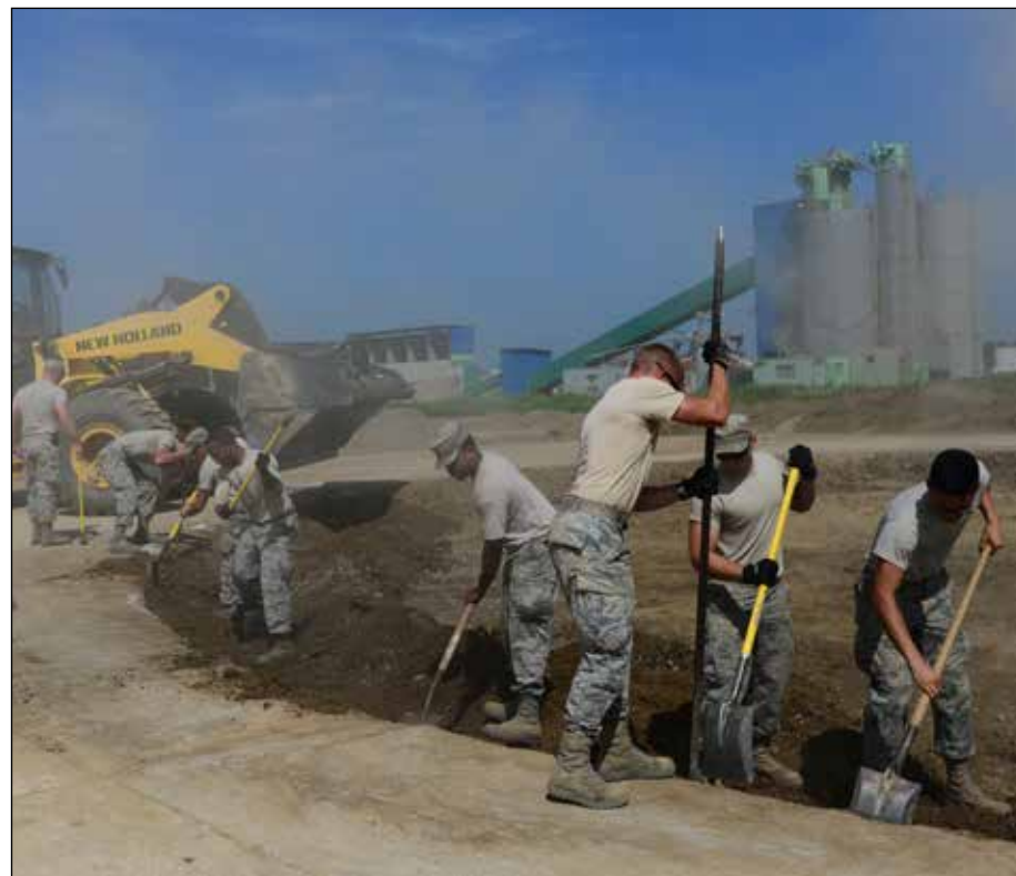
Airmen from the 51st Civil Engineer Squadron pavement and constructions equipment shop, use a combination of heavy equipment and hand tools, to repair a crater during airfield damage repair training at Osan Air Base, Republic of Korea, Aug. 18, 2015. While the overall repair time can vary based on the size, complexity and nature of the situation, the 51st CES toils non-stop to get the base's airfields up and running.
