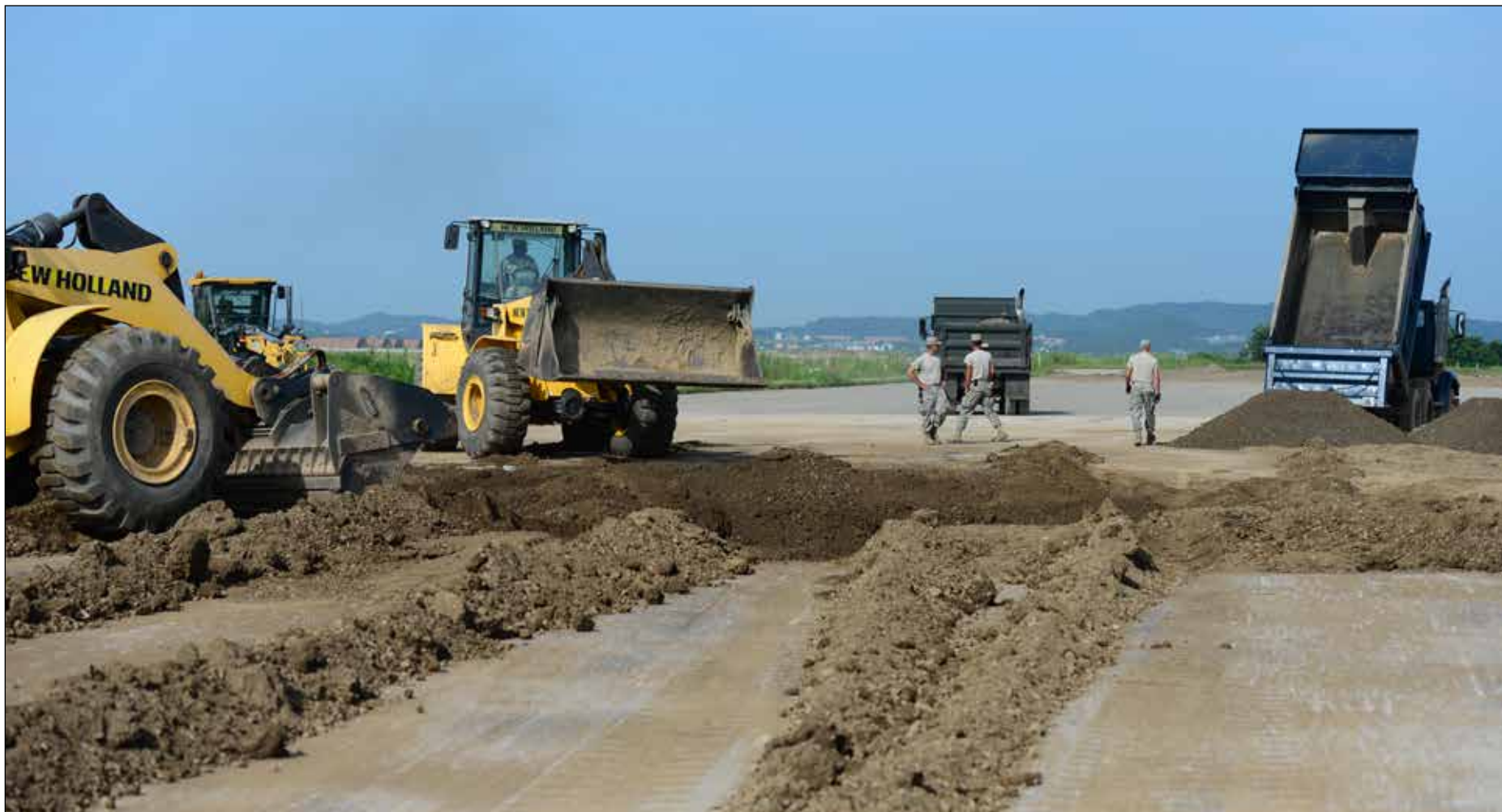
Airmen from the 51st Civil Engineer Squadron pavement and constructions equipment shop, known as the 'Dirt Boyz,' use a method called spoking to repair a crater during airfield damage repair training at Osan Air Base, Republic of Korea, Aug. 18, 2015. Spoking is a term that describes the intricate dance performed by multiple dozers as they work in tandem filling and packing a crater with gravel, dirt and rock. (U.S. Air Force photos by Staff Sgt. Amber Grimm)
