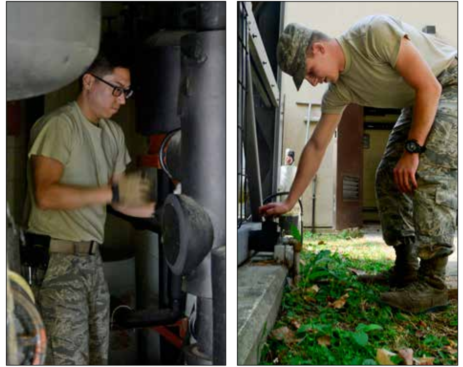
(Left) Staff Sgt. Seung Taek Lee, the 51st Civil Engineer Squadron heating, ventilation and air conditioning technician, empties water from the HVAC system in a building on Osan Air Base, Republic of Korea, Oct. 14, 2015. The water is emptied from the pipes during the No Heat/No Cool season to prevent pipes from freezing in upcoming winter months.
