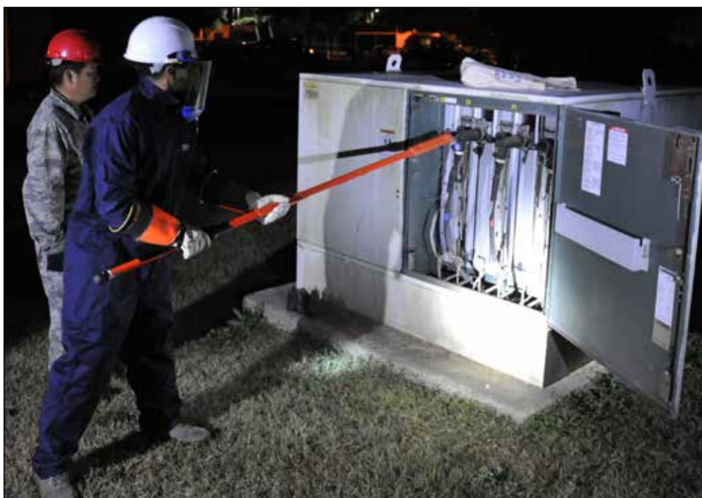
(Above left) Members from the 8th Civil Engineer Squadron replace a transformer during the exercise as part of Beverly Pack 16-1 at Kunsan Air Base, Republic of Korea, Oct. 7, 2015. The exercise tested the ability of Airmen to respond to real world situations. (U.S. Air Force photo by Senior Airman Dustin M. King)
