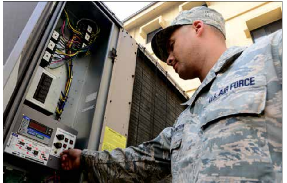
U.S. Air Force Staff Sgt. Aaron Washington, 8th Civil Engineer Squadron heating, ventilation, air conditioning, and refrigeration technician performs a chiller turnoff at a dormitory building for the No Heat/No Cool program at Kunsan Air Base, Republic of Korea, Oct. 22, 2015. The changeover allows HVAC systems to be evaluated and repaired before the heating season begins. (U.S. Air Force photo by Senior Airman Ashley L. Gardner)
