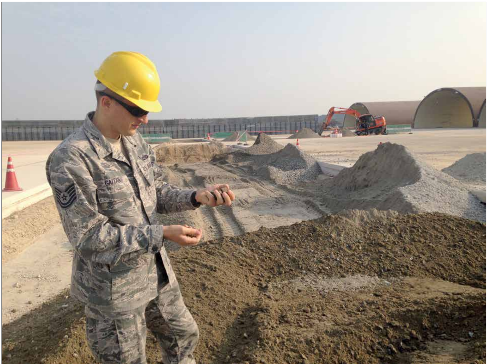
Tech. Sgt. Ioan Gaitan, 607th Materiel Maintenance Squadron, noncommissioned officer in charge of engineering support, inspects aggregate brought on site for an airfield project at Suwon Air Base, Republic of Korea. His job encompasses managing multi-million-dollar contracts and supporting over 600 tenant soldiers living and operating out of the facilities that the Air Force maintains at Suwon AB. Gaitan was recently selected for Officer Training School building on an exemplary enlisted career, one he couldn't have imagined when nine years ago he was randomly selected for a diversity immigrant visa allowing him to leave his home country of Romania and live, study and work freely in the United States. (Courtesy photo)
