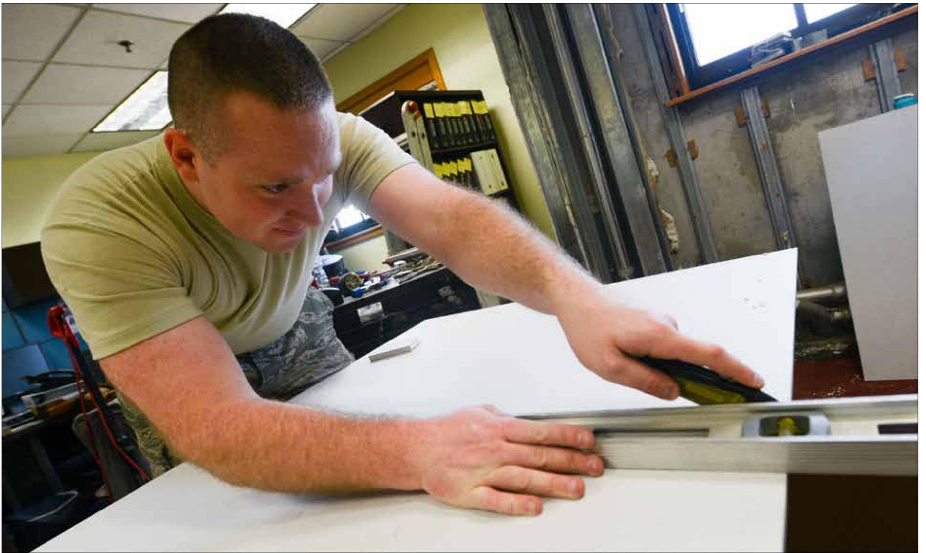
Firefighters from the 51st Civil Engineer Squadron construct a drywall room during construction at Osan Air Base, Republic of Korea, Jan. 14, 2015. The firefighters renovated one of the fire station's rooms to provide better inspection production and customer service from their fire-prevention team. (U.S. Air Force photo by Airman 1st Class Dillian Bamman)
