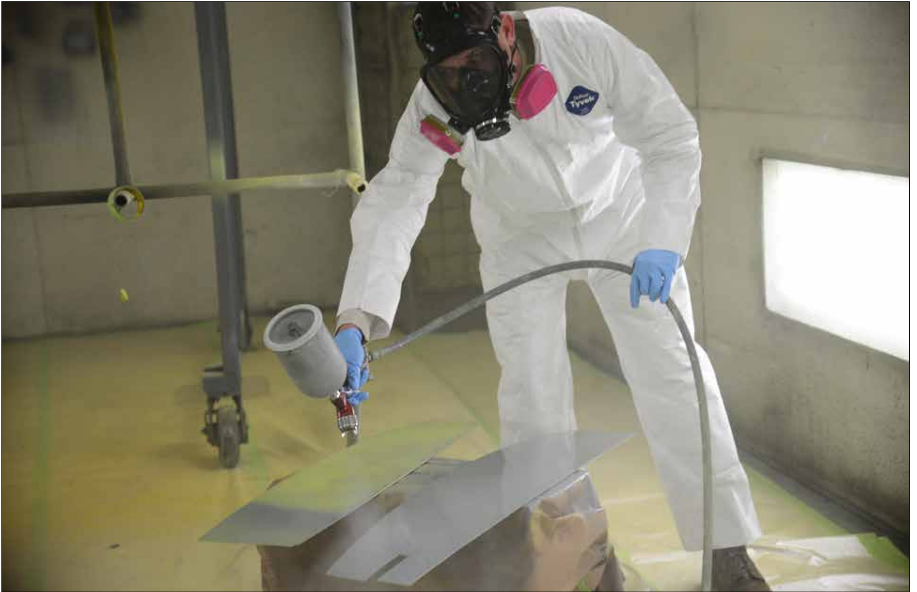
Staff Sgt. Alan Johnson, 51st Maintenance Squadron aircraft structural maintainer, applies a layer of advanced protective paint to aircraft panels at Osan Air Base, Republic of Korea, Jan. 6, 2016. Johnson is a part of the 51st MXS corrosion control shop, commonly known as the "paint barn," where Airmen apply paint touchups to aircraft. (U.S. Air Force photos by Staff Sgt. Amber Grimm)
