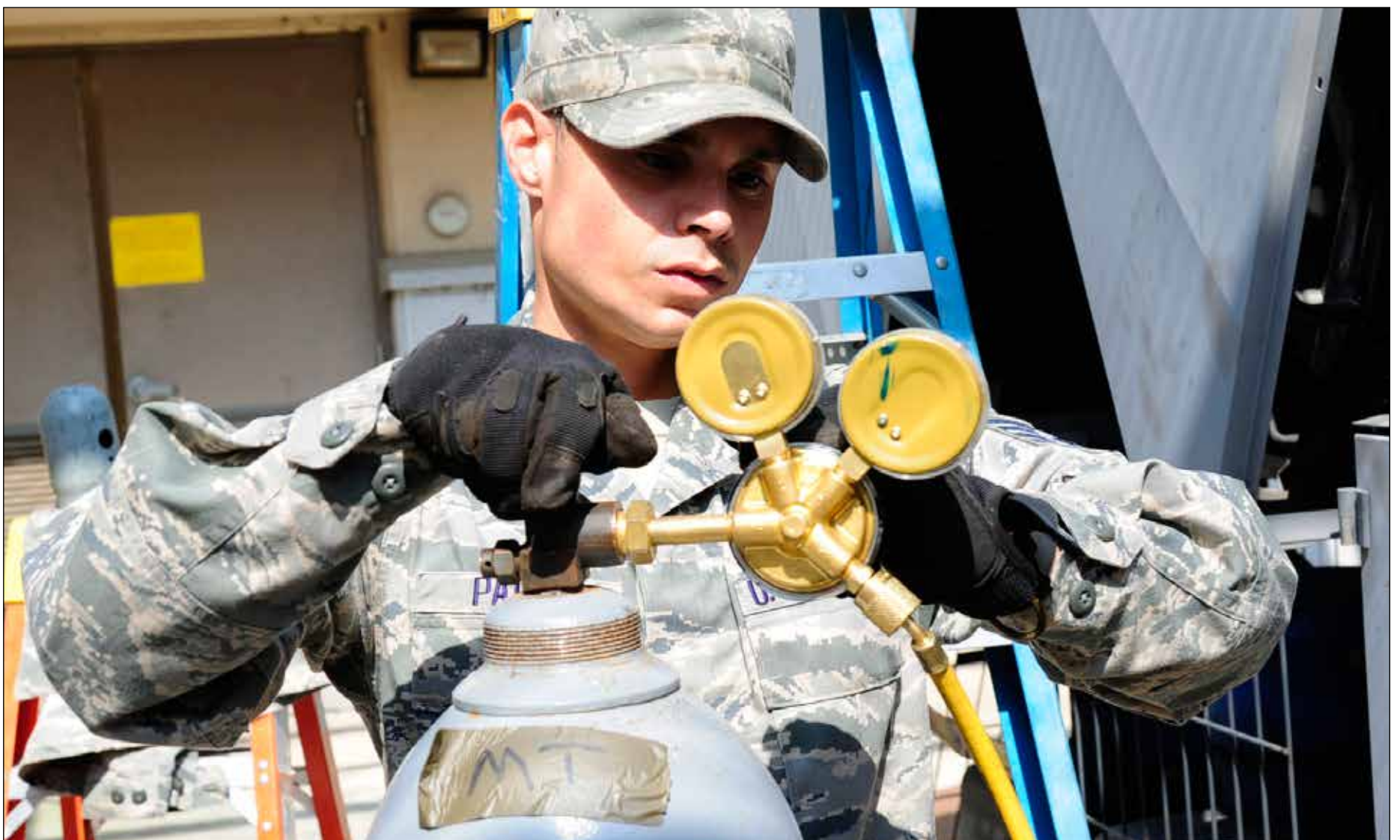
Staff Sgt. Elvis Pabon, 8th Civil Engineer Squadron Heating, Ventilation, and Air Conditioning journeyman, checks for leaks in an air refrigerating machine at the base theater June 7, 2016.
