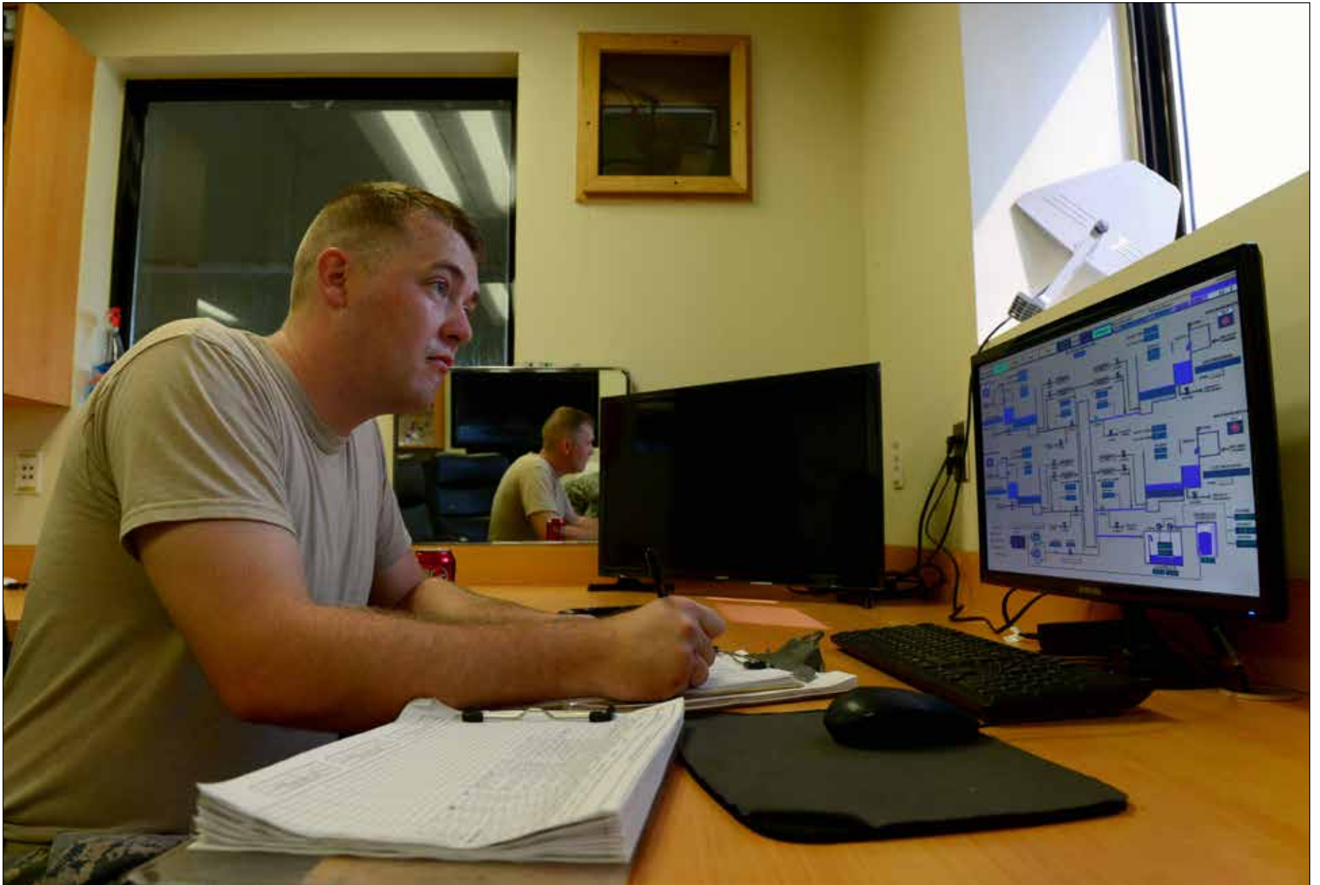
U.S. Air Force Senior Airman Jeremy Robinson, 8th Civil Engineer Squadron Water and Fuels system technician, views the water systems to document pH levels at Kunsan Air Base, Republic of Korea, Aug. 24, 2016. 8th CES Airmen directly maintain 14 water treatment facilities and 24 lift stations throughout the base. (U.S. Air Force photos by Senior Airman Ashley L. Gardner)
