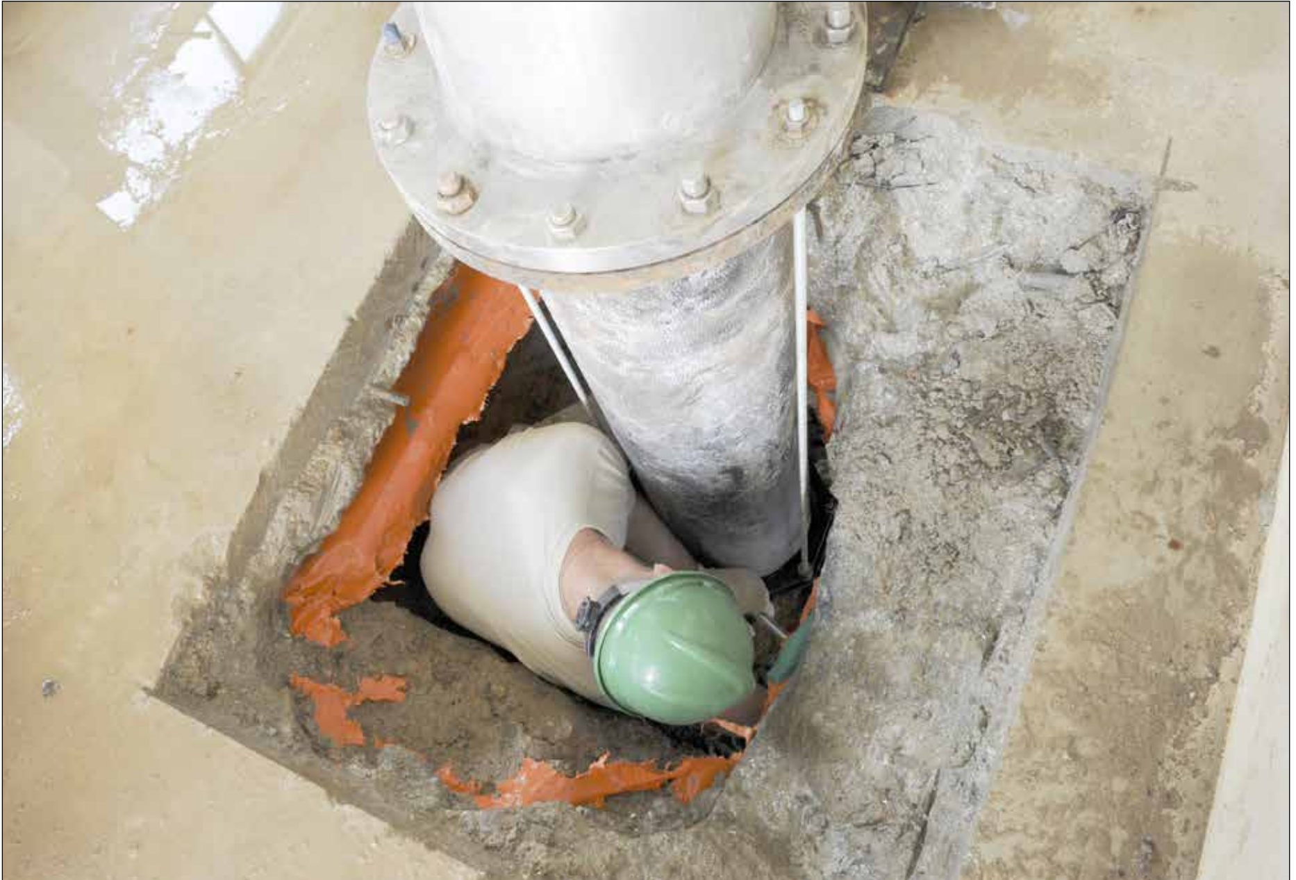
Staff Sgt. Kevin Watters, 8th Civil Engineering Squadron Liquid Fuels noncommissioned officer in charge, replaces a mechanical joint at Kunsan Air Base, Republic of Korea, Oct. 6, 2016. 8th CES members are responsible for maintaining water treatment facilities throughout the base. These facilities provide airmen with potable water so they are continually able to Defend the Base, Accept Follow-On Forces and Take the Fight North. (U.S. Air Force photo by Senior Airman Michael Hunsaker)
