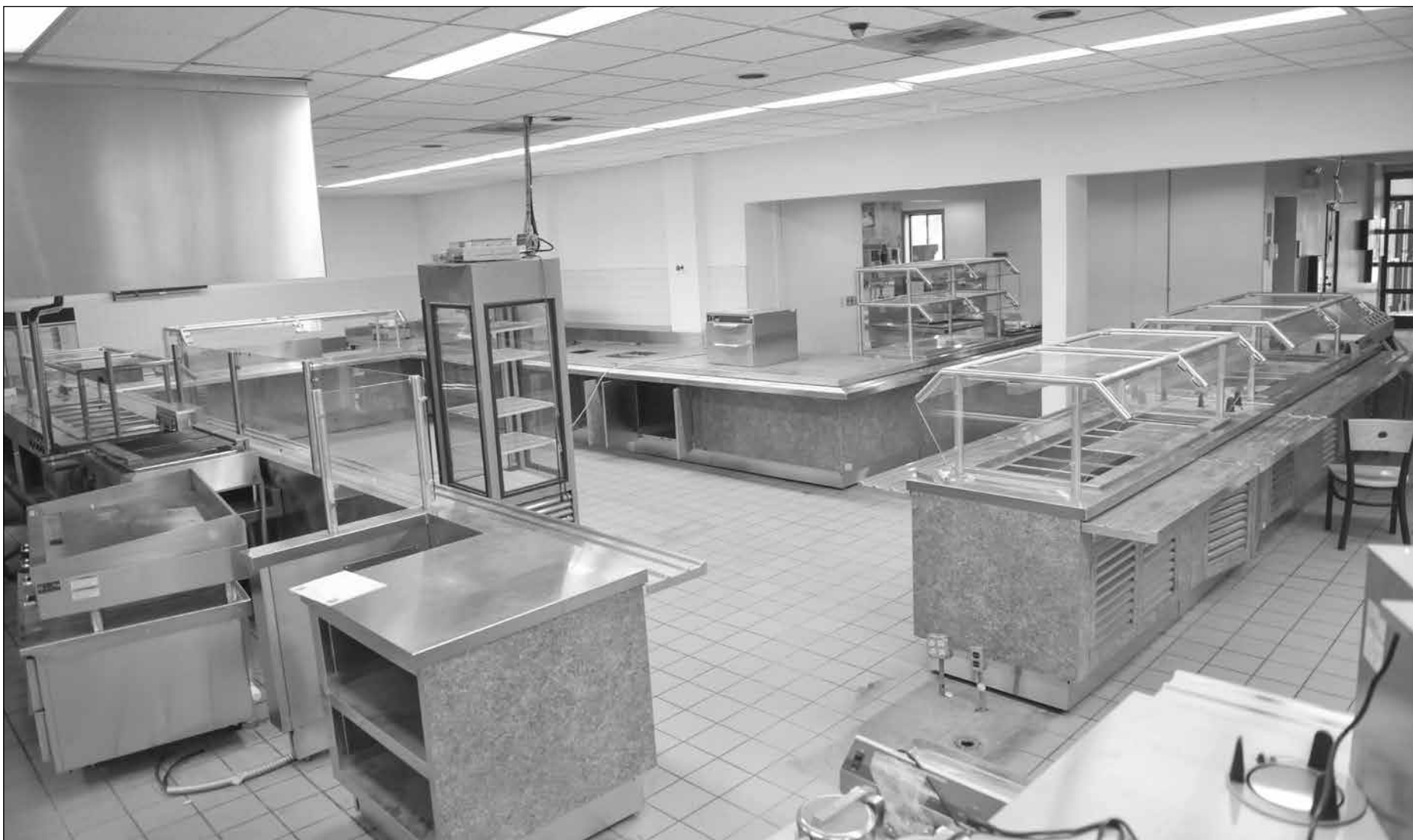
The inside of O'Malley's Dining Facility during construction at Kunsan Air Base, Republic of Korea, Oct. 21, 2016. The dining facility remains closed for renovations and is projected to open back up on Nov. 6, 2016. (U.S. Air Force photo by Senior Airman Colville McFee)
