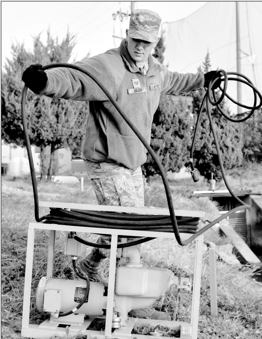
U.S. Air Force Staff Sgt. James Wajda, 51st Civil Engineer Squadron water fuels systems maintenance craftsman, sets up a raw water pump at Osan Air Base, Republic of Korea, Nov. 17, 2016. The pump is used to push water into a filtration system to generate large quantities of drinkable water for the base population. (U.S. Air Force photo by Senior Airman Victor J. Caputo)
