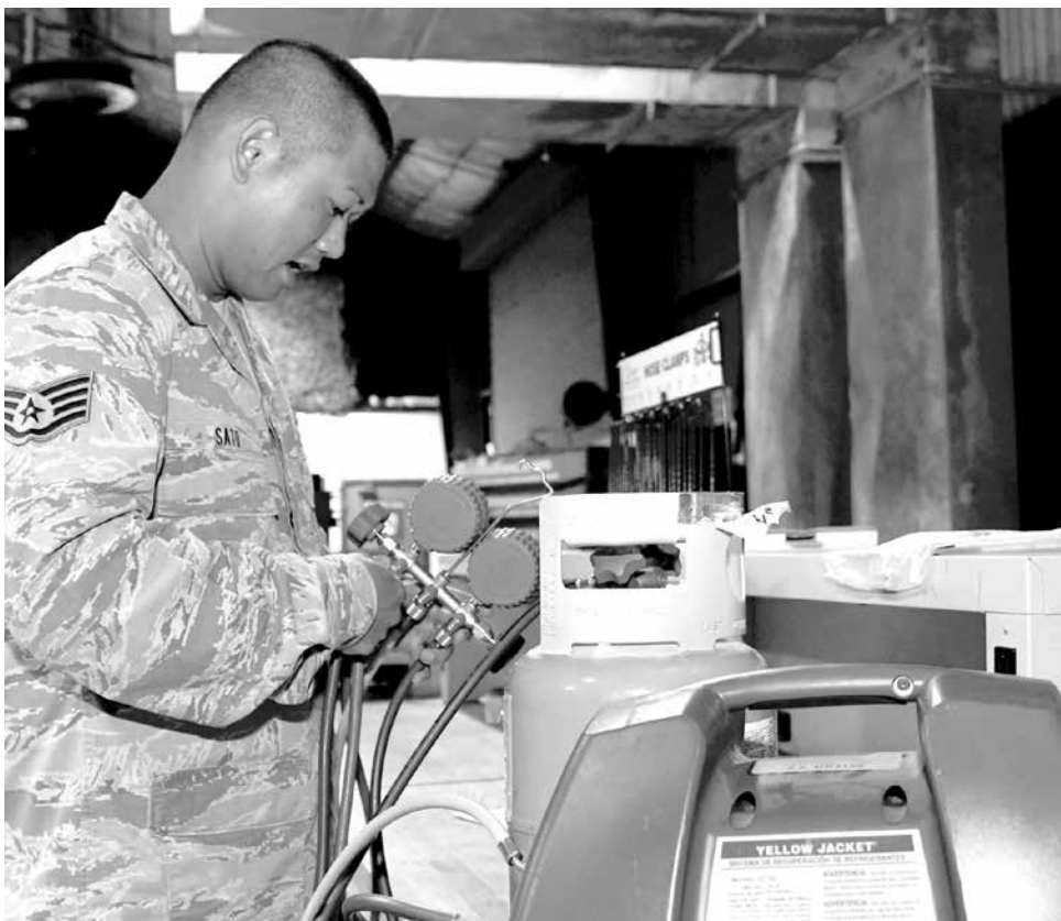
(Above) U.S. Air Force Staff Sgt. Matthew Sato, 51st Civil Engineer Squadron heating, ventilation and air-conditioning technician, works with HVAC gauges at Osan Air Base, Republic of Korea on August 9, 2017. The Osan HVAC shop has 18 active duty military members and 20 civilian contractors that are responsible for almost 600 base facilities. (U.S. Air Force photo by Airman 1st Class Gwendalyn Smith)
