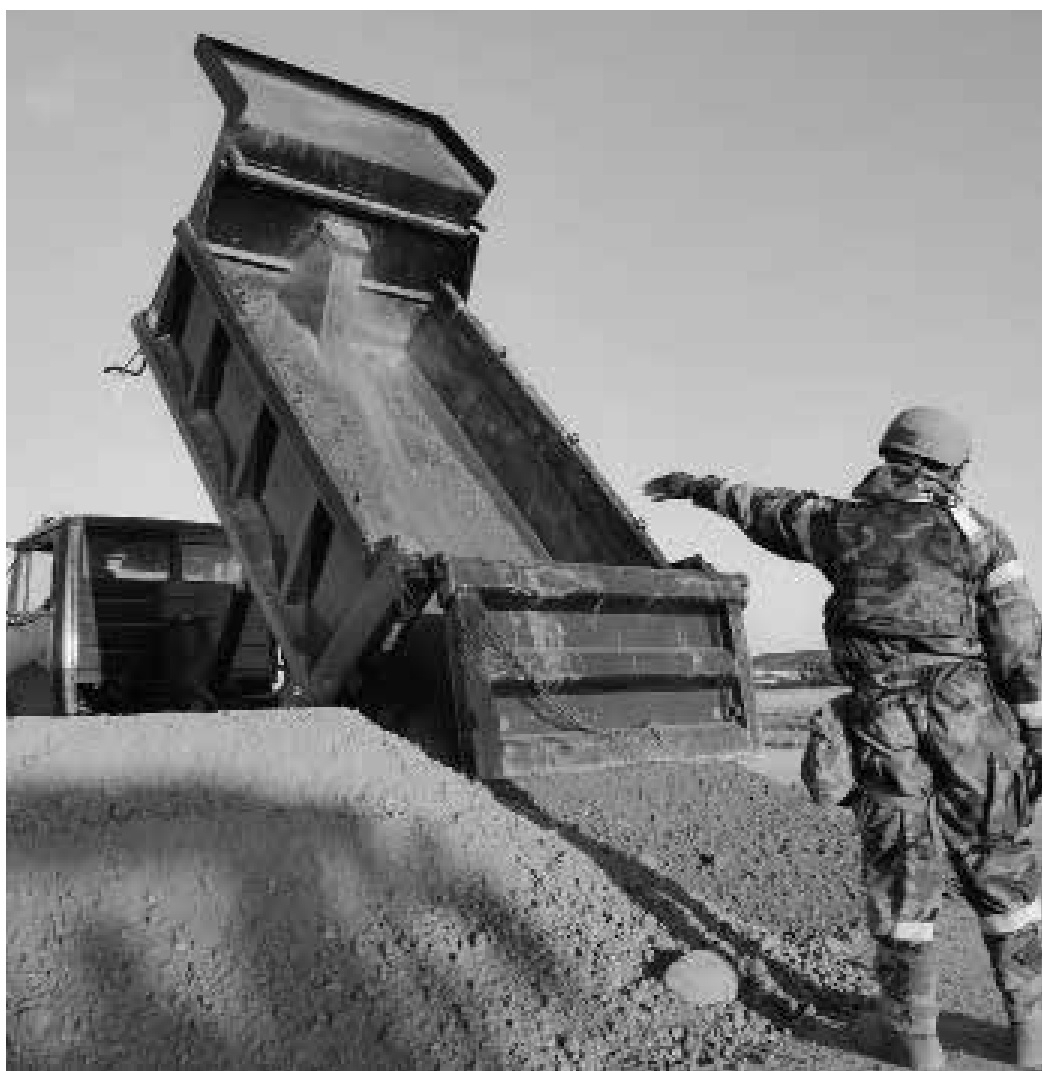
Members of the 51st Civil Engineer Squadron respond to a simulated flightline crater during Exercise Beverly Herd 17-3 at Osan Air Base, Republic of Korea, September 20, 2017. During an attack the civil engineers would fill in the crater and compact it, once it is compact enough a structure is built to go over it. (U.S. Air Force photo by Airman 1st Class Gwendalyn Smith)
