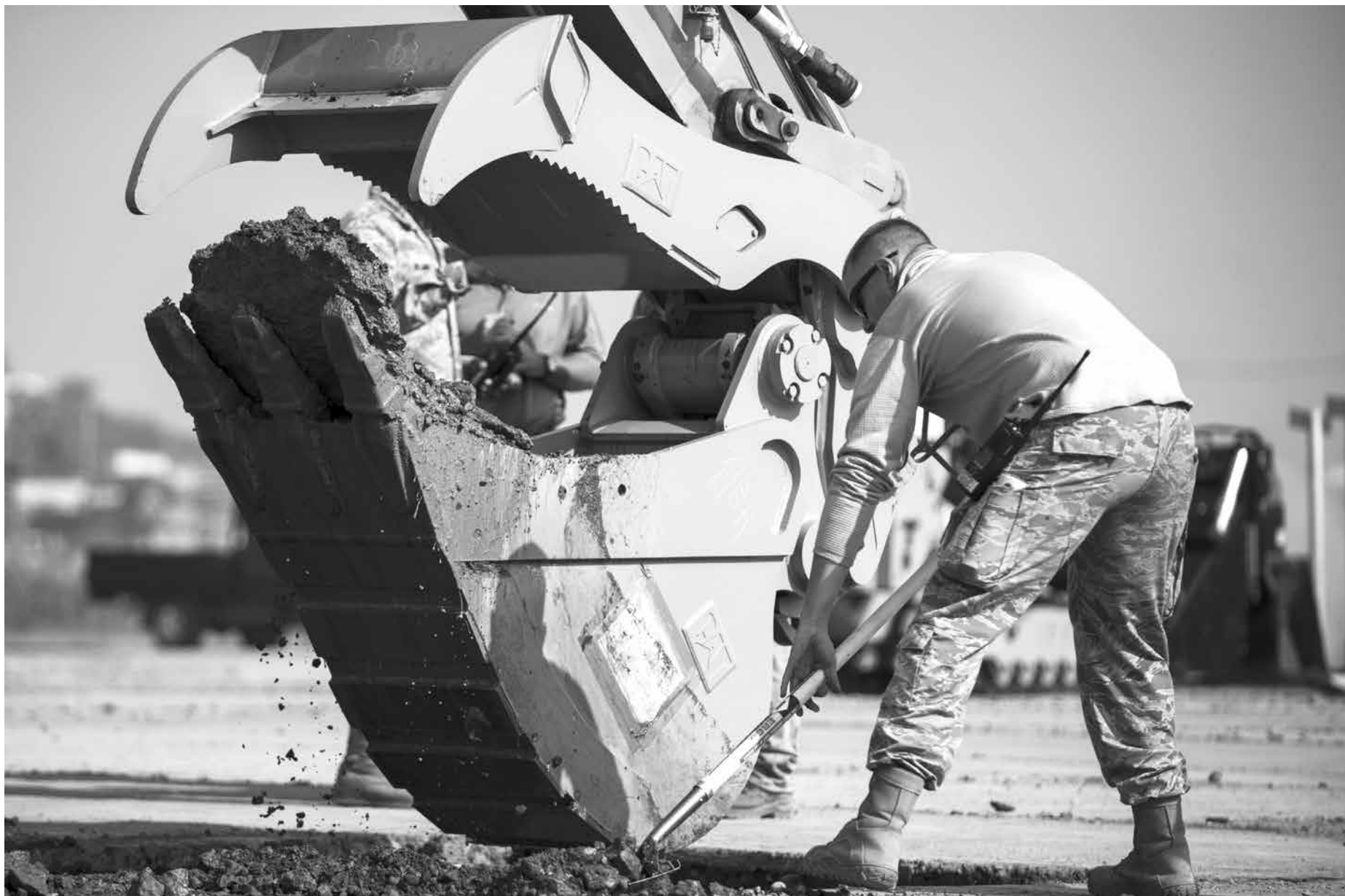
U.S. Air Force Senior Airman Kyle Gibson, 8th Civil Engineer Squadron Water and Fuel Systems Maintenance journeyman, helps to clear debris during rapid airfield damage repair training at Kunsan Air Base, Oct. 25, 2017. The new RADR process was developed by the Air Force Civil Engineer Center to repair damaged airfields at a faster pace. (U.S. Air Force photo by Staff Sgt. Victoria H. Taylor)
