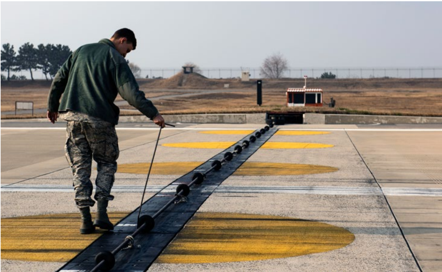
U.S. Air Force Airman 1st Class Zane Mammon, 8th Civil Engineer Squadron electrical power production specialist, adjusts a rubber support on a barrier arresting kit at Kunsan Air Base, Republic of Korea, Dec. 19, 2018. Aircraft arresting systems are designed to safely stop an aircraft that's experiencing an in-flight emergency and cannot land without causing damage. (U.S. Air Force photo by Senior Airman Stefan Alvarez) ◀
