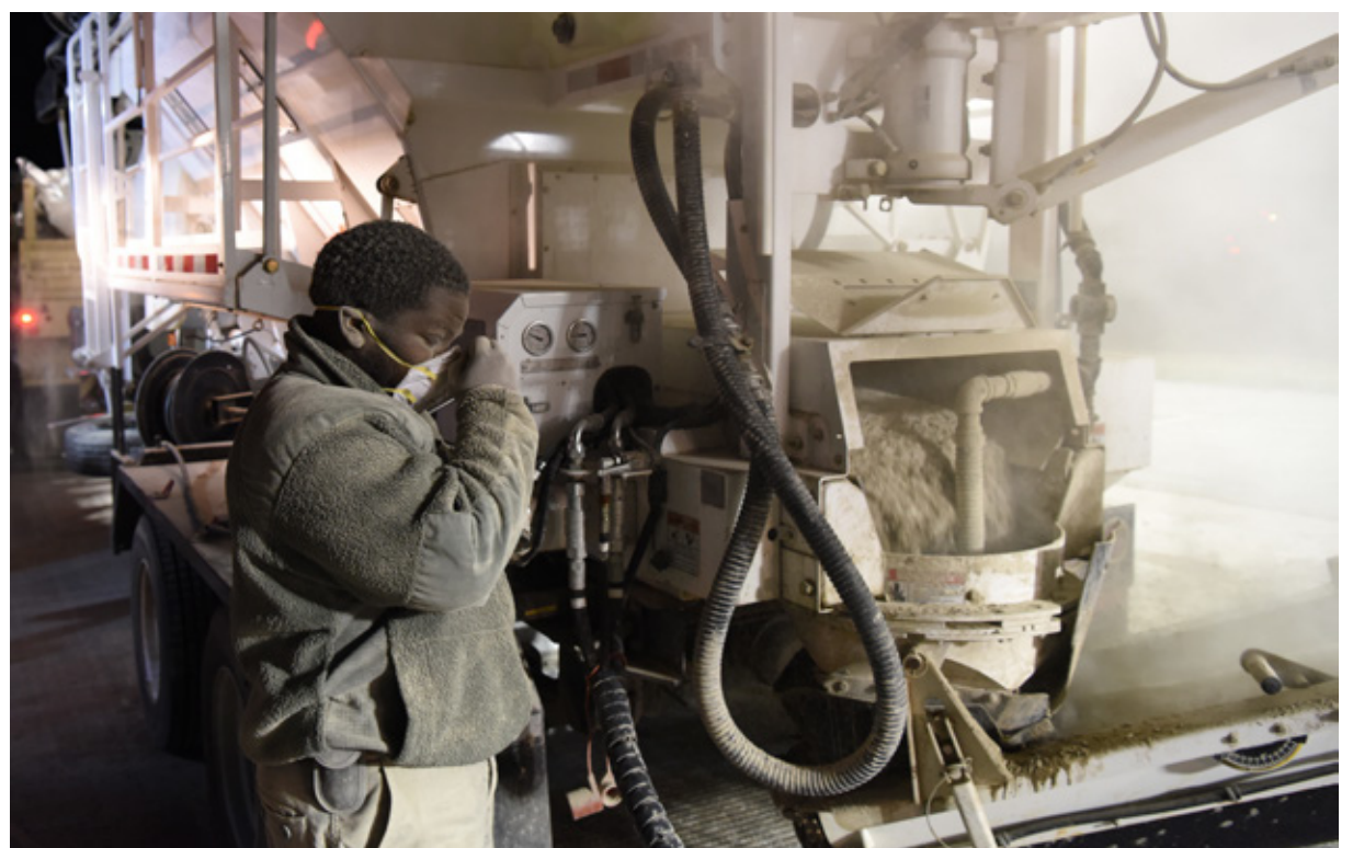
U.S. Air Force Staff Sergeant Christopher Leonard, 8th Civil Engineer Squadron pavement and construction equipment journeyman, adjusts his face mask while pouring cement at Kunsan Air Base, Republic of Korea, May 2, 2019. The 8th Civil Engineer Squadron dug out a corroded pipe that caused a rupture and restored the site in less than 24 hours. (U.S. Air Force photo by Staff Sgt. Joshua Edwards)
