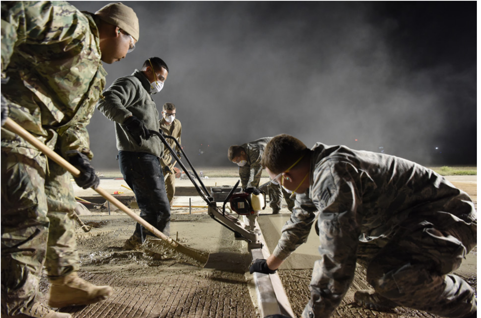
U.S. Air Force 8th Civil Engineer Squadron members smooth concrete on the flight line at Kunsan Air Base, Republic of Korea, May 2, 2019. The 8th CES applied rapid airfield damage repair methods to fix a rupture that caused damage to the flight line. (U.S. Air Force photo by Staff Sgt. Joshua Edwards)
