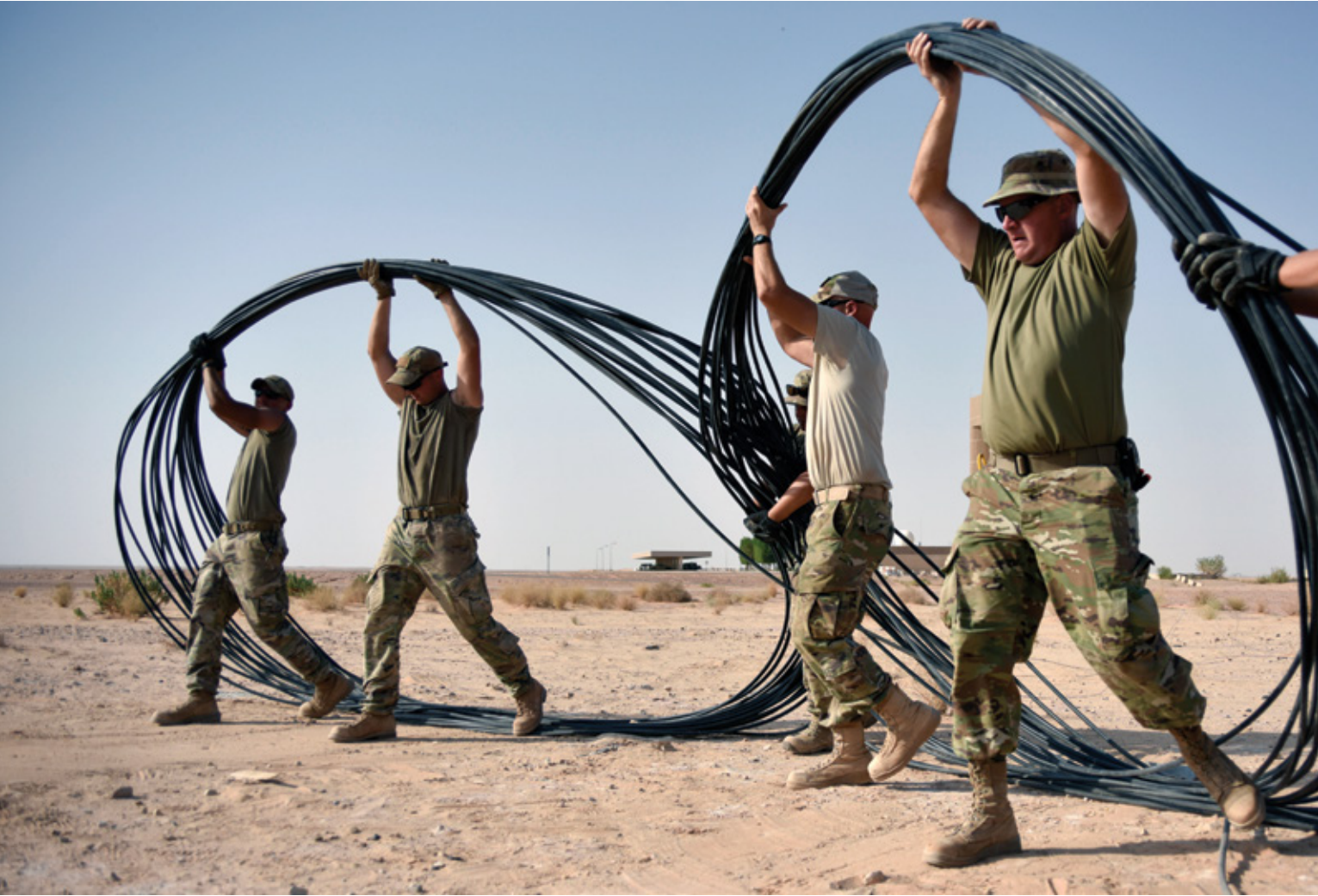
A irmen with the 210th Engineering Installation Squadron move fiber-optic cable into place prior to running it to the next access point at Prince Sultan Air Base, Saudi Arabia, Nov. 5, 2019. The 210th EIS is installing approximately 120,000 feet of cable, increasing the capability, reliability and security of the networks at Prince Sultan AB. (U.S. Air Force photo by Tech. Sgt. John Wilkes) ◀
