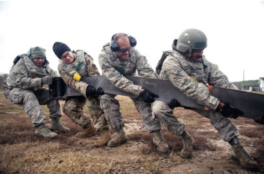
A irmen assigned to the 203rd RED HORSE Squadron, Virginia Air National Guard, set up a mobile aircraft arresting cable during a four-day field training exercise, Nov. 16, 2019, at State Military Reservation, Virginia Beach, Va. RED HORSE stands for Rapid Engineer Deployable Heavy Operations Repair Squadron Engineers. (U.S. Air National Guard photo by Senior Airman Bryan Myhr) ▲
