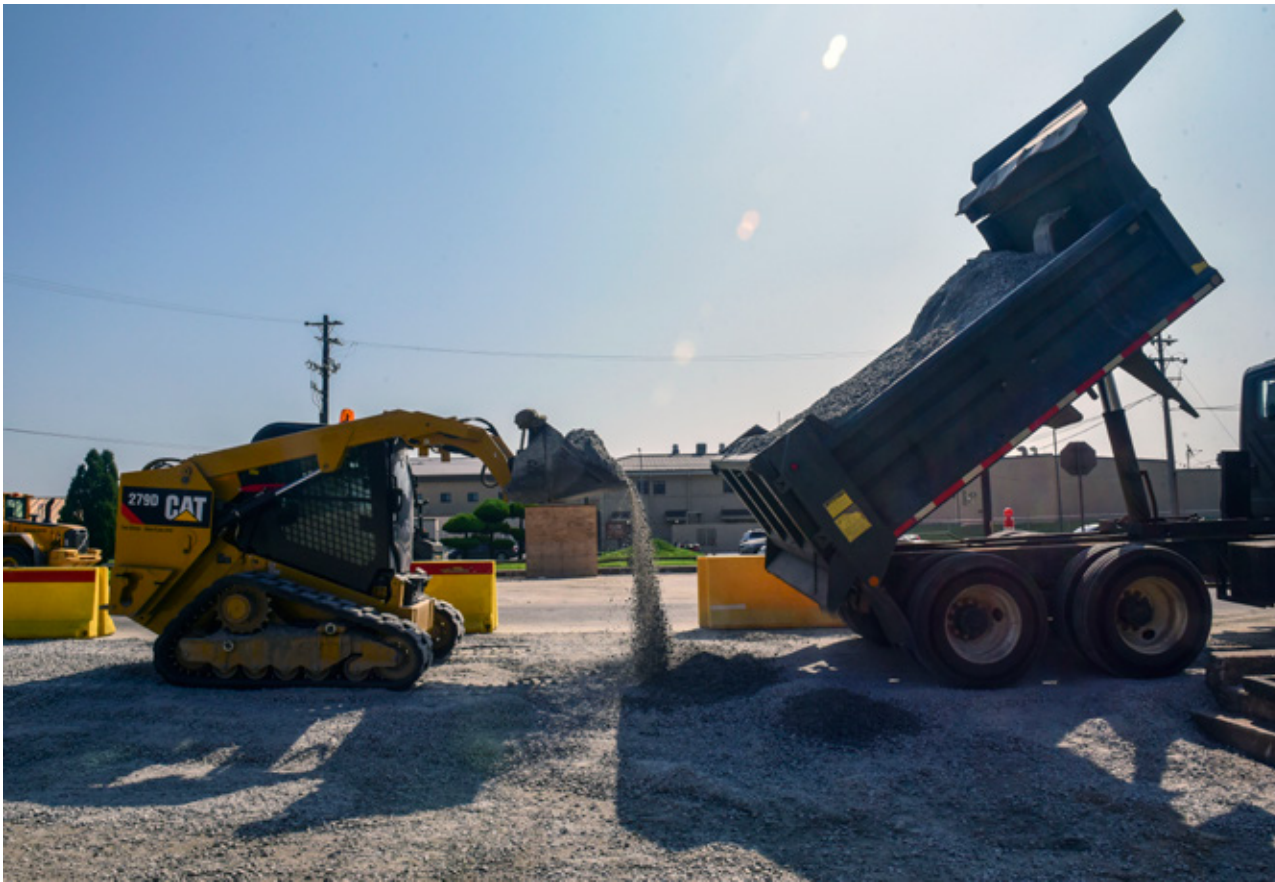
Senior Airman Harold McIntyre, 8th Civil Engineer Squadron heavy equipment and pavement personnel, removes gravel from a dump truck at Kunsan Air Base, Republic of Korea, Aug. 23, 2020. Repairing landscaping, drainage, fencing, concrete and asphalt and even snow removal are just a few of the capabilities that the 8th Civil Engineer Squadron provides when maintaining the infrastructure. (U.S. Air Force photo by Senior Airman Jessica Blair) ◀
