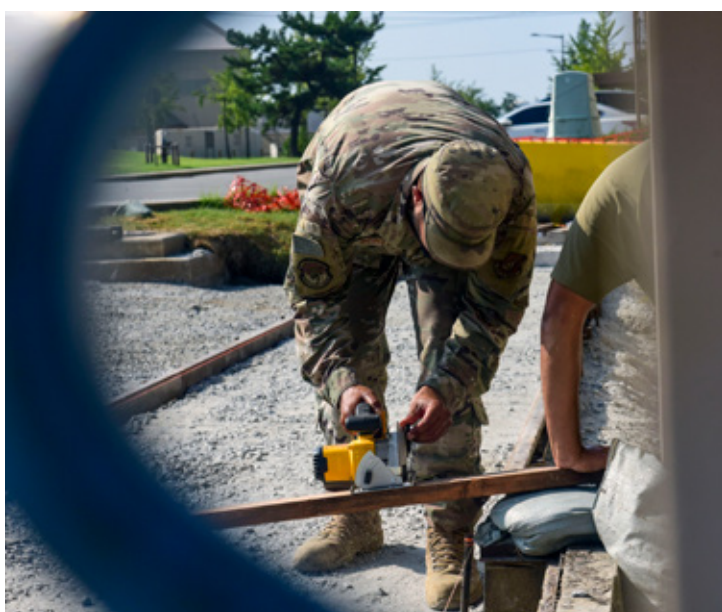
Senior Airman Harold McIntyre, 8th Civil Engineer Squadron heavy equipment and pavement personnel, cuts wood with a saw at Kunsan Air Base, Republic of Korea, Aug. 23, 2020. Heavy equipment and pavement personnel do everything from operating heavy construction equipment to detonating explosives when maintaining the facilities used on base every day. (U.S. Air Force photo by Senior Airman Jessica Blair) ▲
