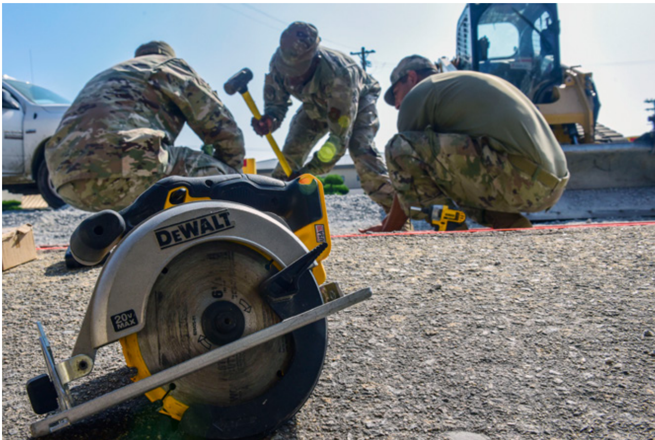
Staff Sgt. Jimmy Noriega, Senior Airmen Harold McIntyre, and Pryde Nchamukong, 8th Civil Engineer Squadron heavy equipment and pavement personnel, drive metal stakes into the ground during sidewalk construction at Kunsan Air Base, Republic of Korea, Aug. 23, 2020. The Dirt Boys construct runways and airfields in remote locations in addition to maintaining facilities already in use. (U.S. Air Force photo by Senior Airman Jessica Blair) ◀
