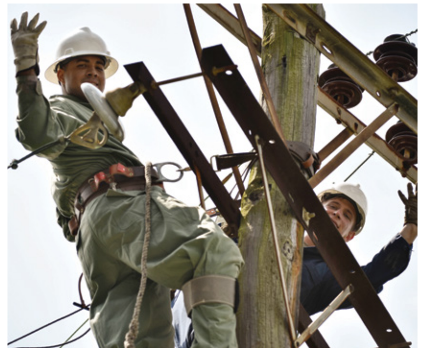
Tech. Sgt. Chaz Lineberger and Senior Airman Cody McCormick 8th Civil Engineer Squadron electrical systems technicians, prepare a line for reattachment in response to Typhoon Maysak at Kunsan Air Base, Republic of Korea, Sept. 3, 2020. The heavy equipment and pavement shop assisted the 8th CES electrical systems shop in response to the damage caused by Typhoon Maysak. (U.S. Air Force photo by Senior Airman Mya M. Crosby) ▲
