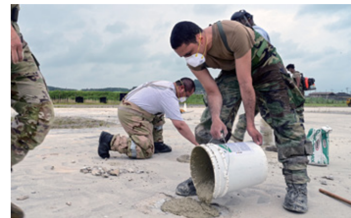
U.S. Air Force Senior Airman Gabriel Vivas, 8th Civil Engineer Squadron heating, ventilation and air conditioning spall team member, pours concrete quick mix into a hole during exercise Beverly Sentinel 25-3 at Kunsan Air Base, Republic of Korea, Aug. 6, 2025. The hole was created on a simulated flightline area to allow the Red Devils to practice Rapid Airfield Damage Repair (RA/DR). ▲
