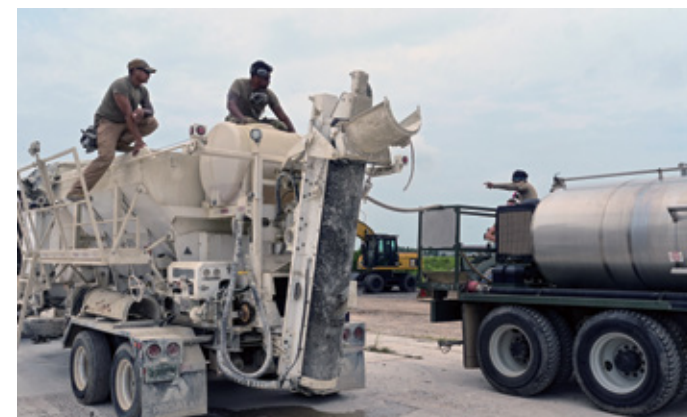
U.S. Air Force Senior Airman Gabriel Vivas, 8th Civil Engineer Squadron heating, ventilation and air conditioning spall team member, pours concrete quick mix into a hole during exercise Beverly Sentinel 25-3 at Kunsan Air Base, Republic of Korea, Aug. 6, 2025. The hole was created on a simulated flightline area to allow the Red Devils to practice Rapid Airfield Damage Repair (RA/DR). ▲
