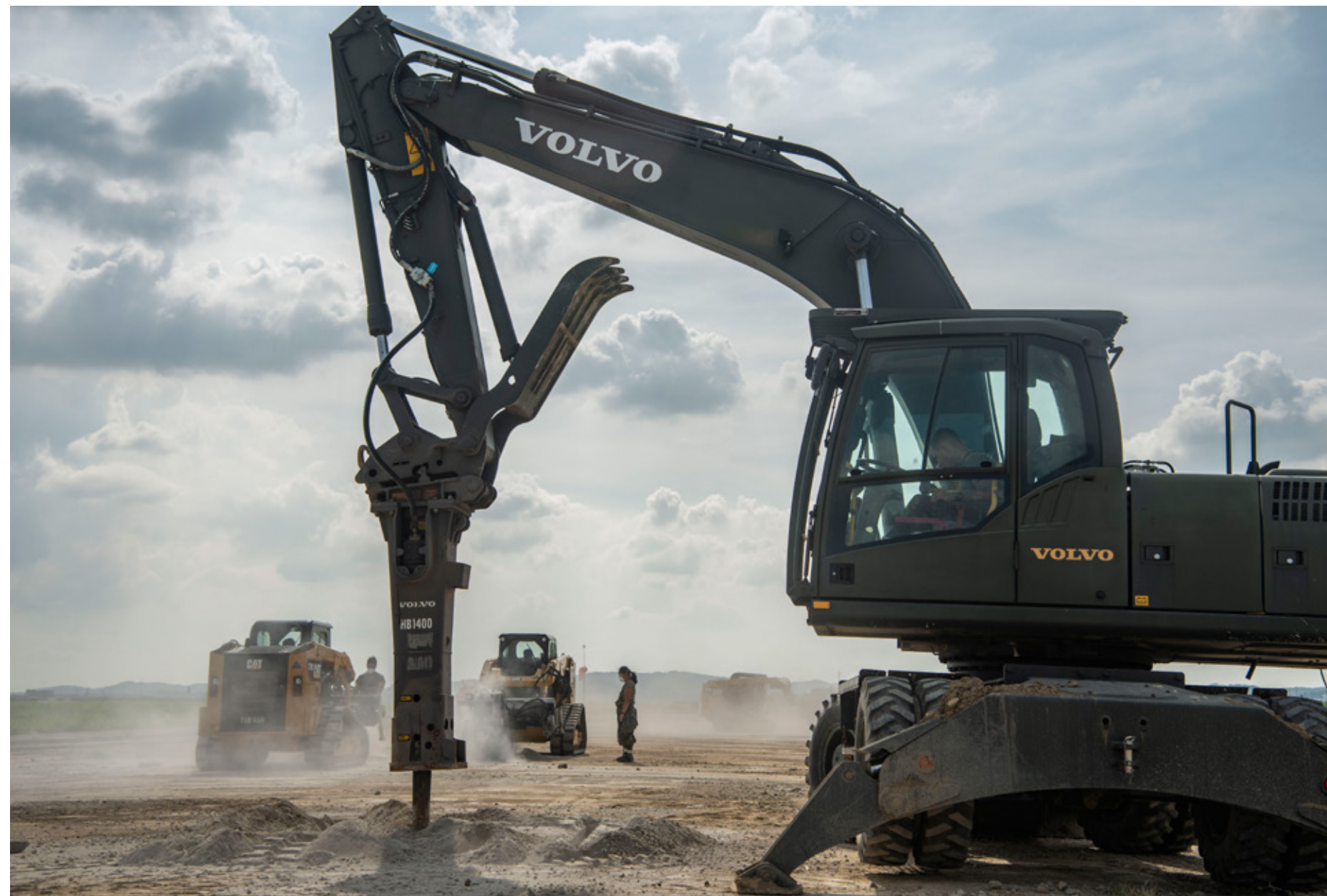
A U.S. Air Force Airman assigned to the 51st Civil Engineer Squadron uses a vehicle mounted jackhammer to break up portions of unusable concrete to conduct rapid airfield damage repair during exercise Ulchi Freedom Shield 25 at Osan Air Base, Republic of Korea, Aug. 20, 2025. RADR consists of assessing the damage, separating unusable concrete by cutting it out, fracturing the unusable section to be excavated and then filling the void with the appropriate material. (U.S. Air Force photo by Staff Sgt. Jason W. Cochran) ▲
