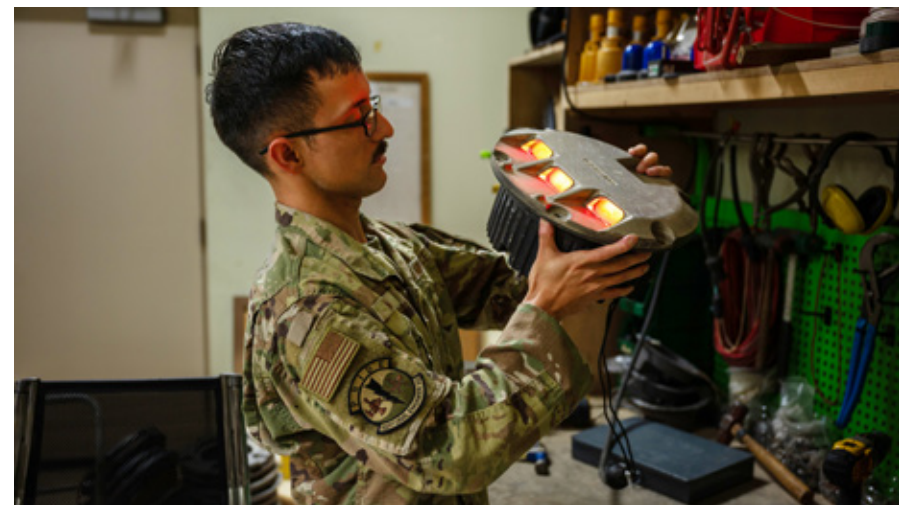
U.S. Air Force Staff Sgt. Jose Medina, 51st Civil Engineer Squadron electrical systems craftsman, inspects an approach light at Osan Air Base, Republic of Korea, Sept. 3, 2025. Medina is tasked with maintaining and certifying the operability of the approach lights, ensuring pilots know whether to land, stop, or align with the runway depending on the color that is displayed. ▲
