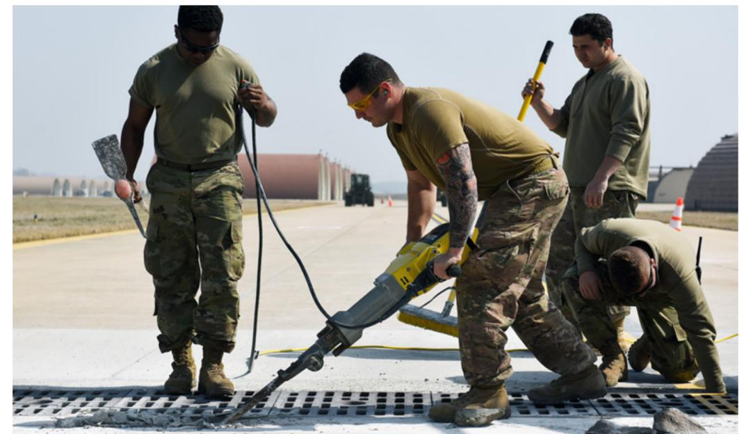
Airman 1st Class Chase Pavlenko, 8th Civil Engineer Squadron pavements and heavy equipment operator, uses a K-12 saw to cut out cracked concrete on a taxiway at Kunsan Air Base, Republic of Korea, March 23, 2021. The 8th CES is replacing failed concrete on the flightline to prevent foreign object debris hazards. (U.S. Air Force photo by Senior Airman Suzie Plotnikov) ▼
